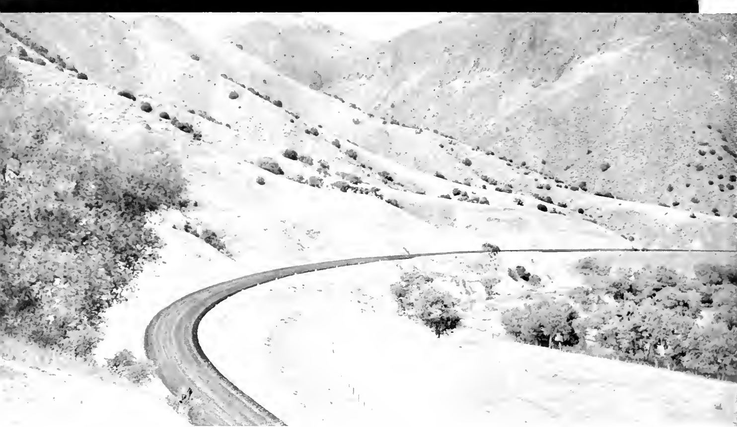
New surfaced road through Warthan Canyon swings high above creek bed avoiding a dangerous crossing of ravaging stream
